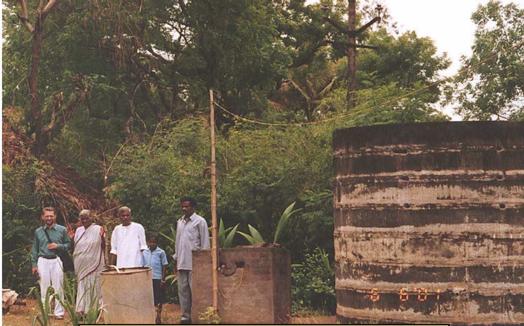
Missionary Centre Project. Water storage, pump and bore well.
